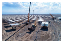
Heliostats Lifting
