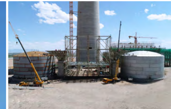
Salt Tank & Thermal Exchange Platform Construction
